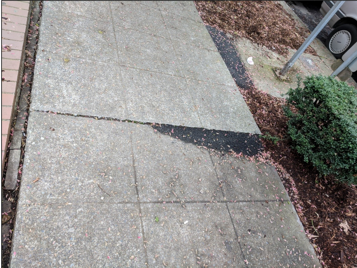
Figure 3: Existing Conditions - Asphalt Shim
