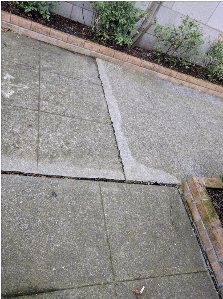
Figure 4: Existing Conditions - Beveling
