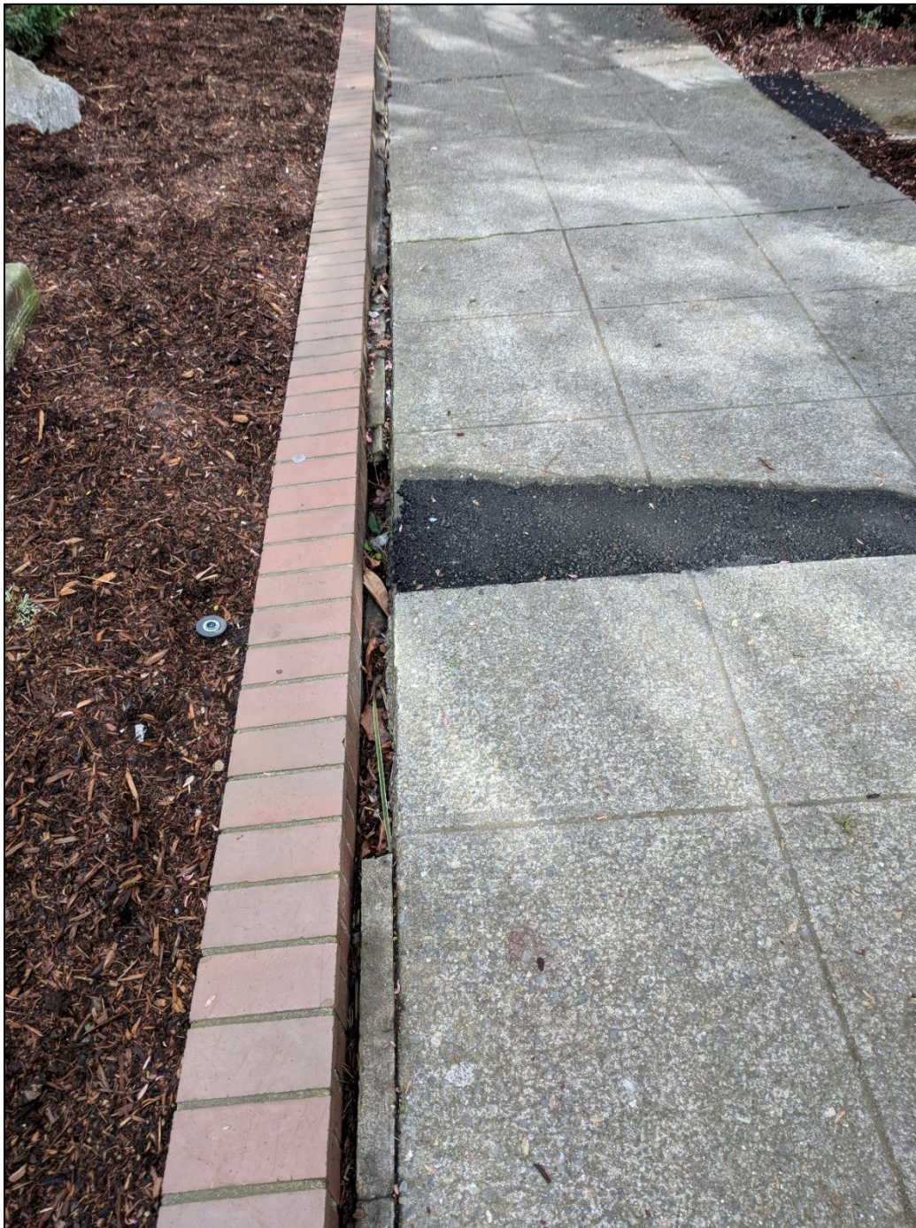
Figure 2: Existing Conditions - Asphalt Shim
