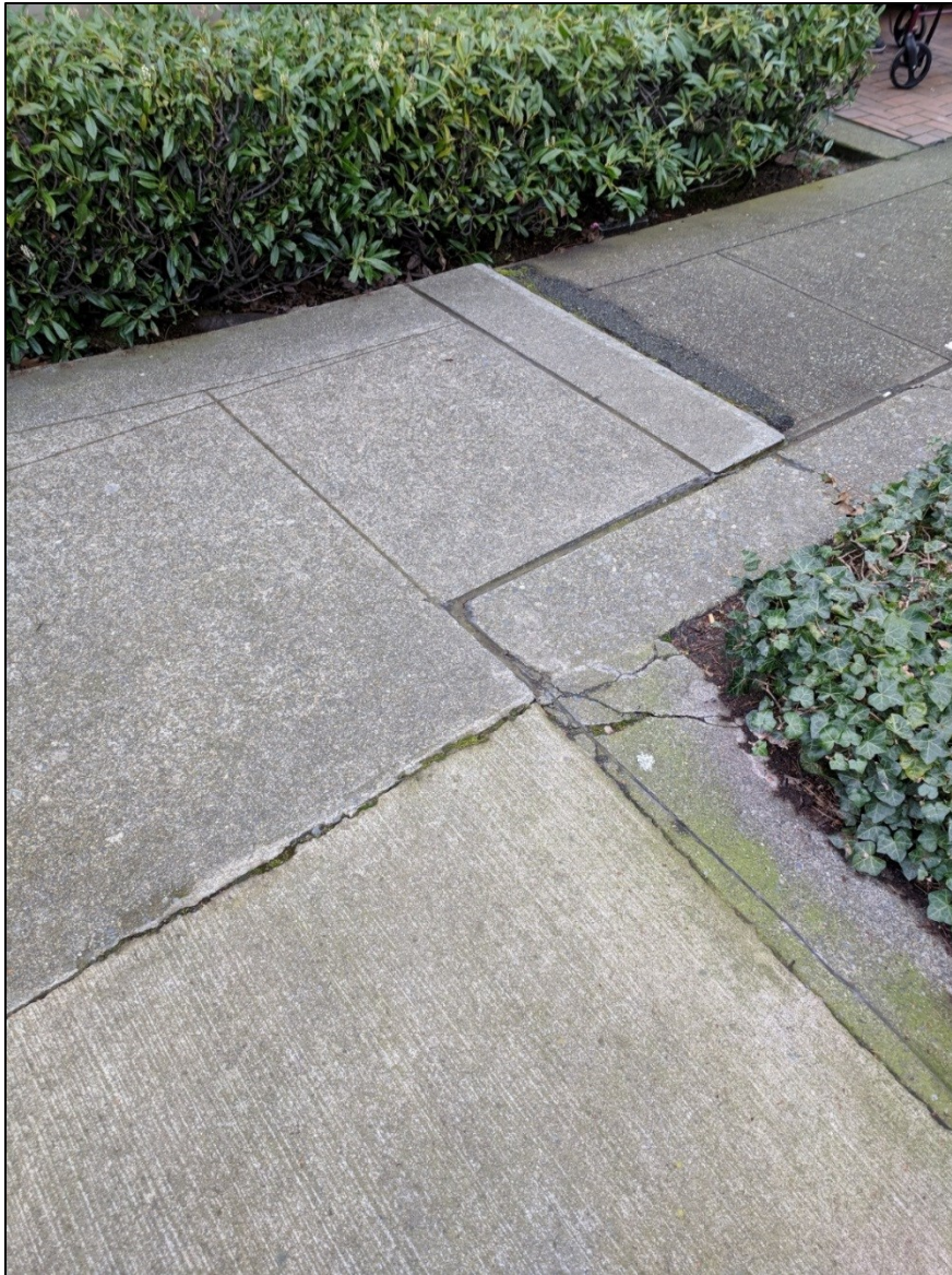
Figure 1: Existing Condition - Asphalt Shim
